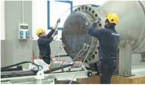
Anchoring to the shell 1
